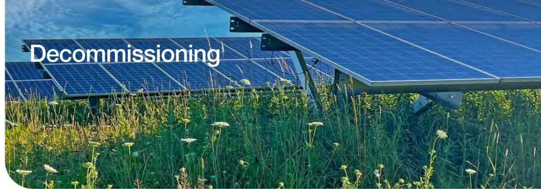
Like any electrical waste, solar panels need to be disposed of responsibly and safely. Solar panels are up to 99% recyclable, and the major panel components including the glass, aluminium and copper can all be recovered.
